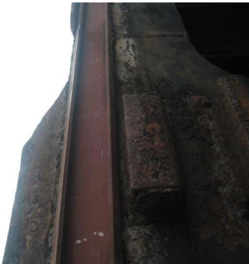
Rubber channel fitted and adjusted.
