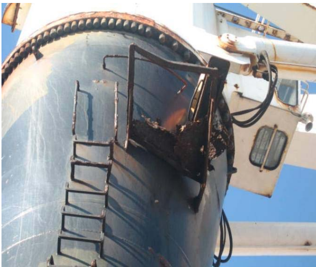
Crane No1 with destroyed platforms
