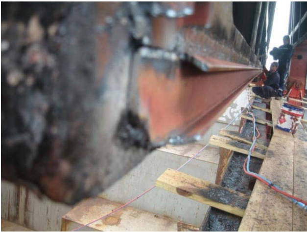
Rubber channel fitted and adjusted At ends.
