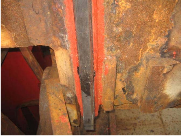
Rubber packing replacement at side
