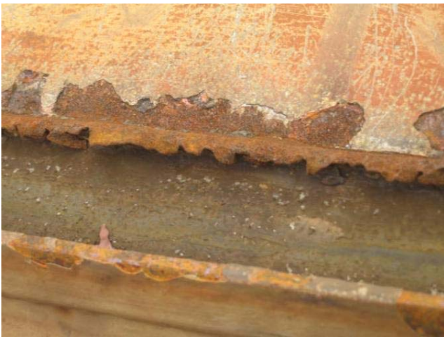
Cross joint rubber channel as found Is totally wasted.
