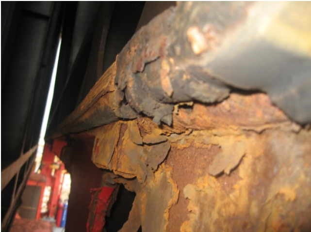
Internal view of packing in Poor condition as found.
