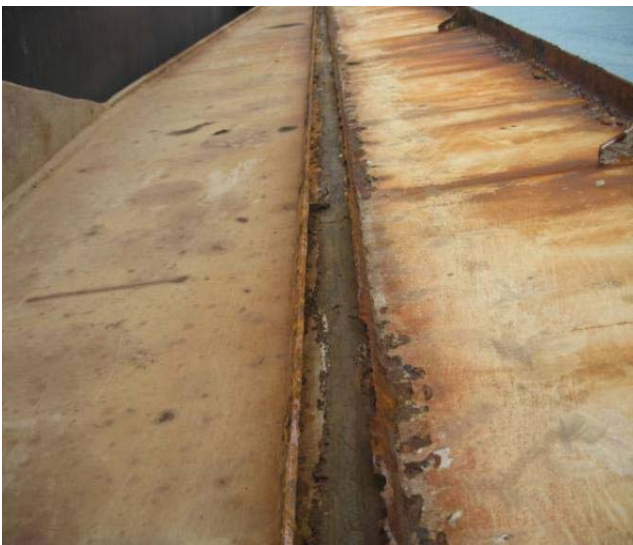
General view of channel as found Totally wasted.
