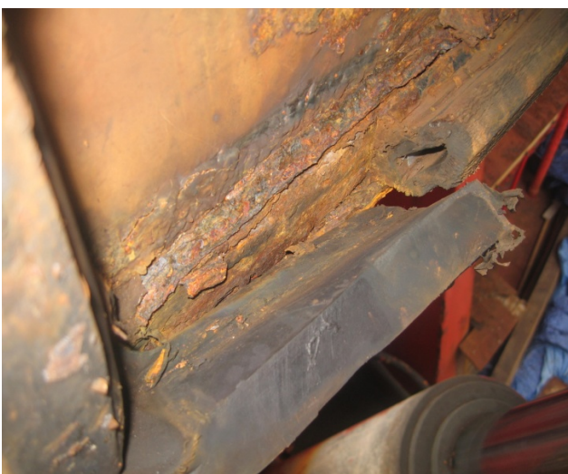
Broken rubber packing as Found
