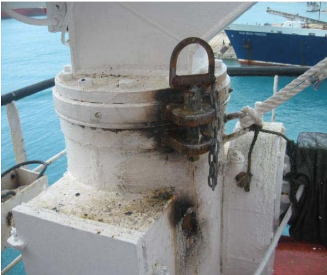
Safety pin fabricated and installed at Provision cranes port/stbd.
