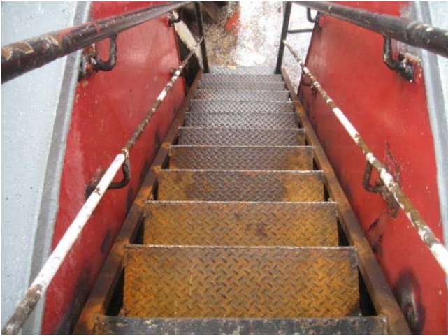
New steps installed at port External accommodation ladder
