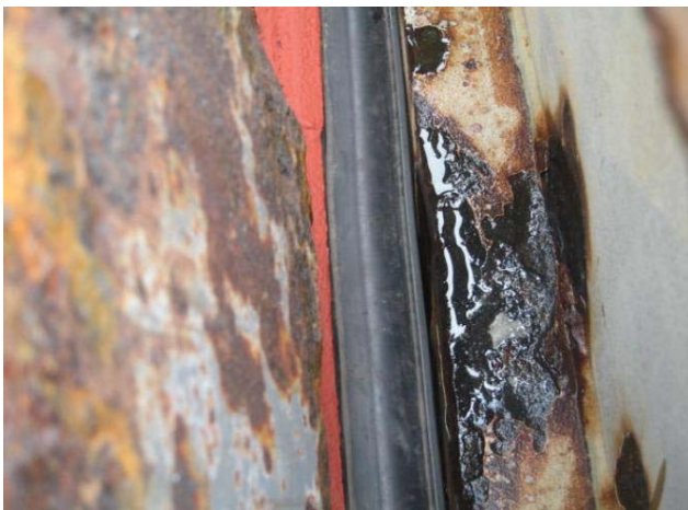
Cross joint as found with big gap Between packing and flat Compression.
