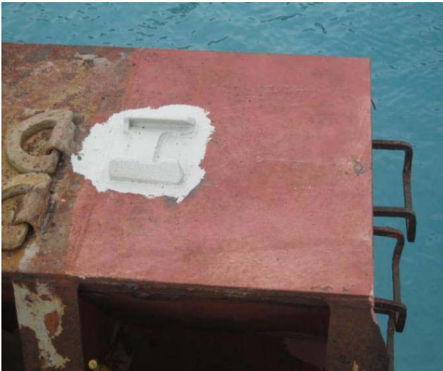
Above repaired and container fittings Adjusting and installed
