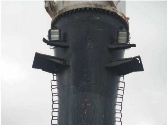
Destroyed platforms of crane no2.
