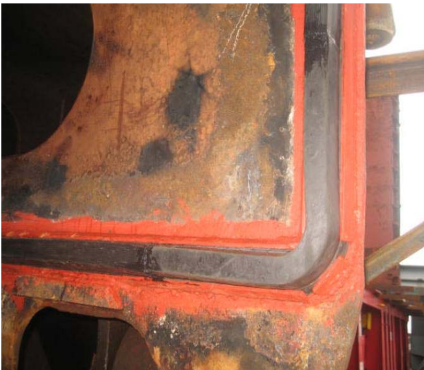
Corner packing replacement
