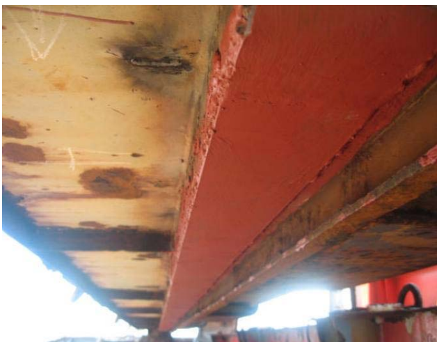
Flat compression as placed and Adjusted.
