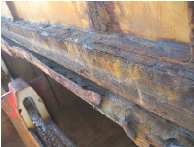
Compression flat and drain channel In poor condition as found
