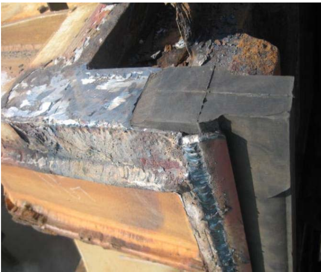
Another view of fitting with Modification on channel too.
